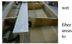
Apply two  $\frac{1}{2}$ " beads of milled fiber along the entire length of the spar. These beads should be approximately 1" in from the edge of the wing spar.
