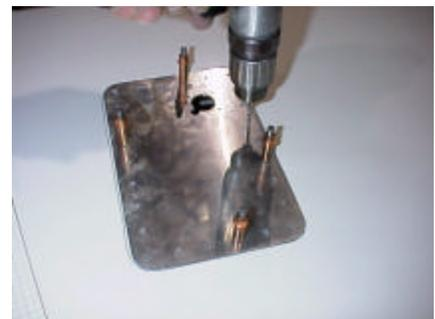
**Step 3. Install backing plate.**
