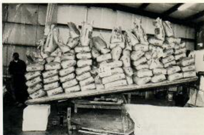
EXPRESS wing was loaded to 11 G's without failure.
